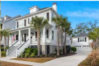
1910 Bellona Street Under Contract for Buyer
