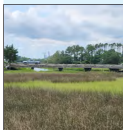
Nowell Creek footbridge construction to begin
